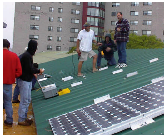
Philadelphia’s Weatherization team solar project
